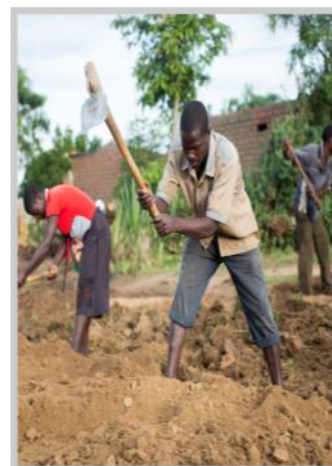
Men at work—Roads project in Dedza
