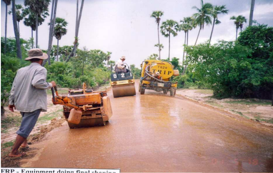
FRP - Equipment doing final leveling
